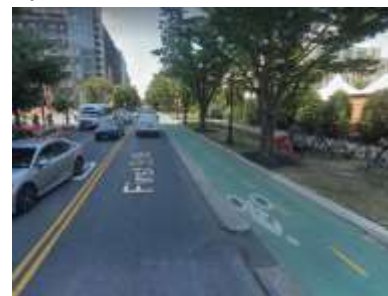
Cycletrack (1st St. NE, D.C.)
