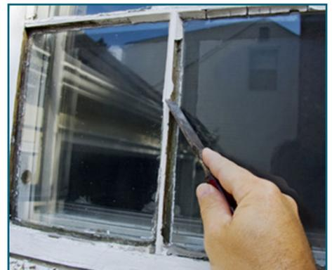
**Old paint and caulk**, including surrounding substrate such as brick, masonry, cinder block, wood, etc., can create dust containing PCBs during renovations. Care must be taken during removal of these materials and they must be disposed of properly.
