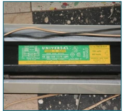
**Fluorescent light ballasts (FLBs)** can contain PCBs and should be removed and disposed of by trained professionals.
