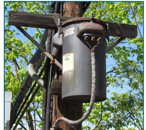
**PCB-contaminated transformers** that contain more than 50 ppm of PCBs are subject to specific EPA regulations. Proper PCB identification labels must be visible near the access and on the transformer itself.
